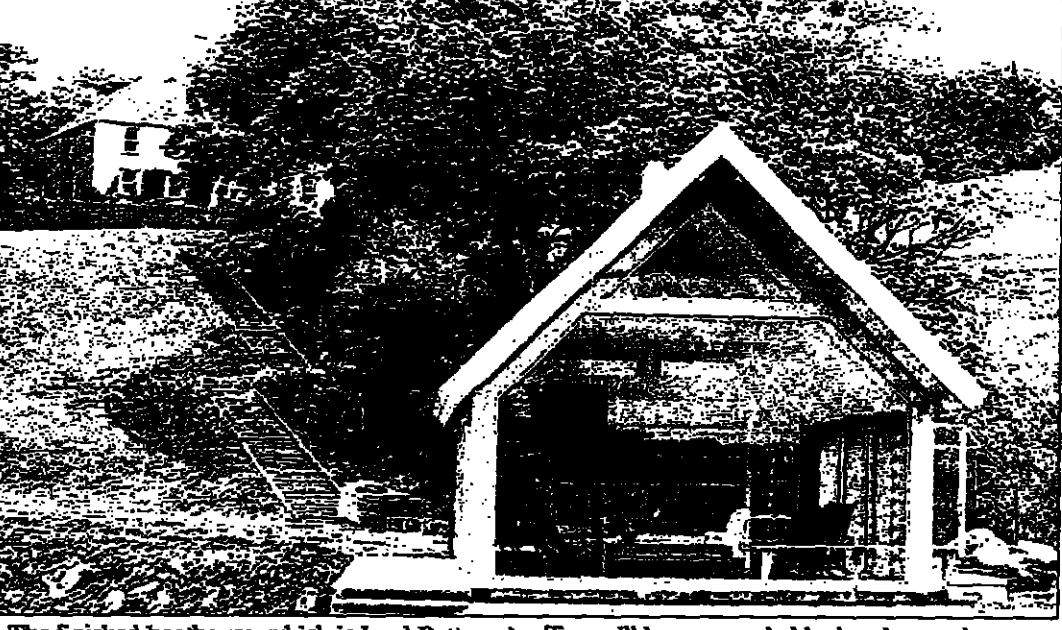
The finished boathouse, which is Lord Putnam's office, will be surrounded by bamboo and acers
